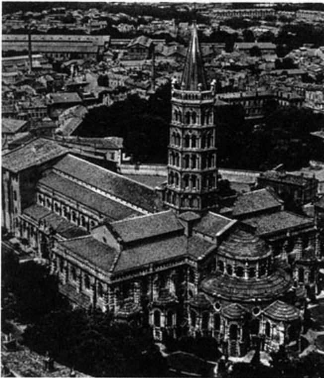
Fig. 3. St.-Sernin, aerial view.
